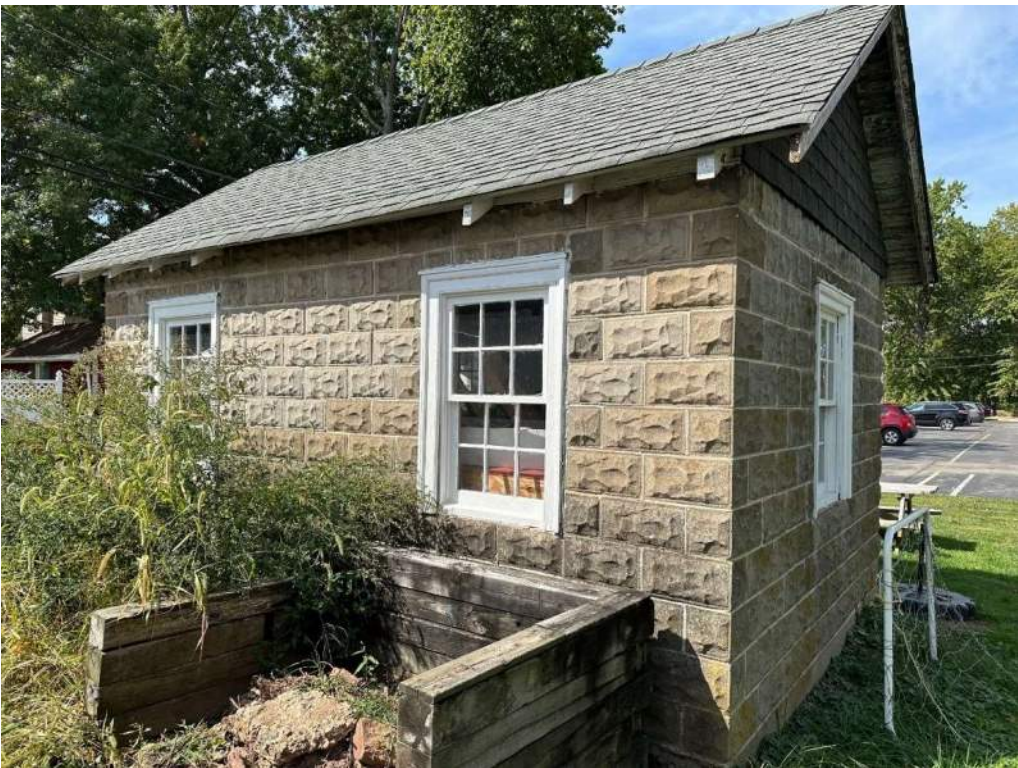
Photograph 4 – Existing Garage (Side)
