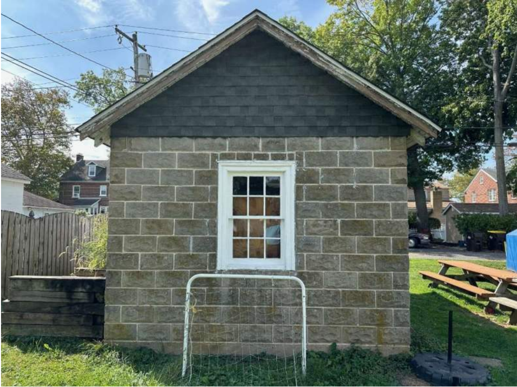
Photograph 3 – Existing Garage (Rear)
