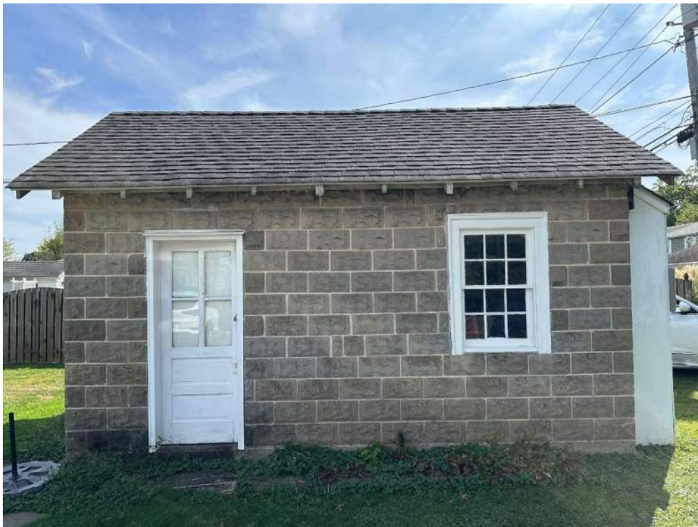
Photograph 2 – Existing Garage (Side)
