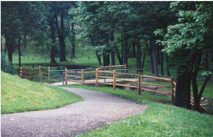
Bridge over Towamencin Creek at Whites Road Park
