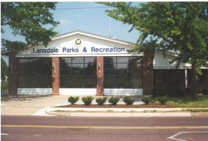
Lansdale Park & Recreation Building , Lansdale Avenue
