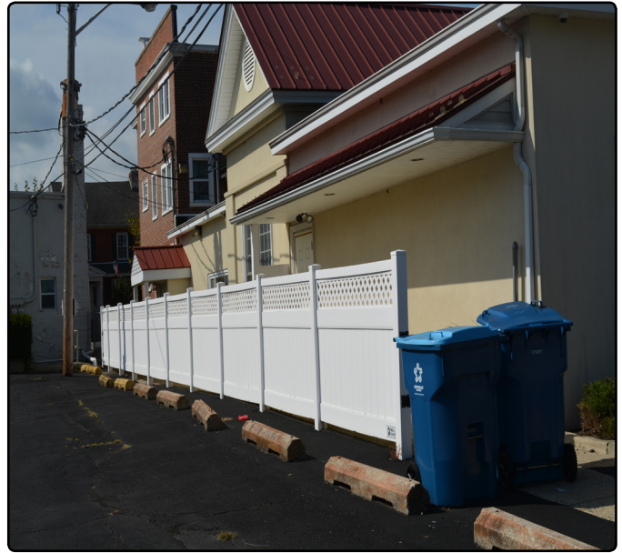
Landscaping and fencing can be used to screen spaces between buildings.
